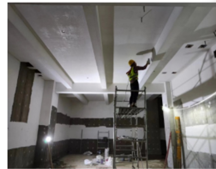
basement plaster work
