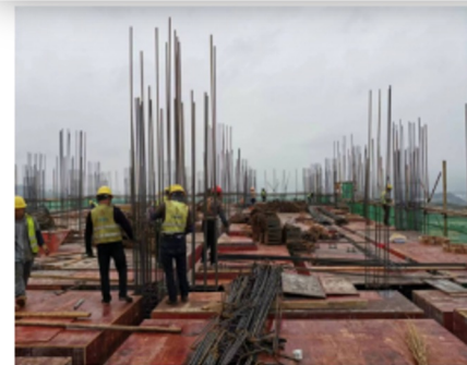
28.4m floor working
