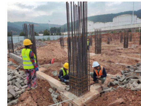
office start foundation brick wall
