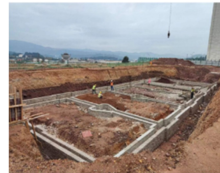
firefighting tank brick form work
