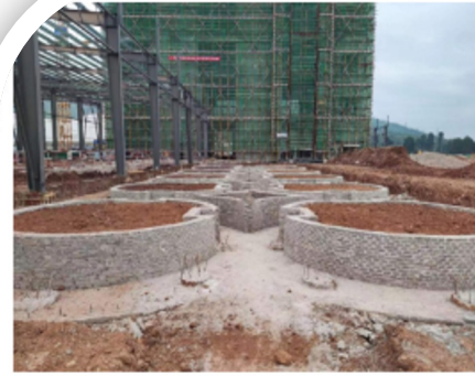
small silo area
