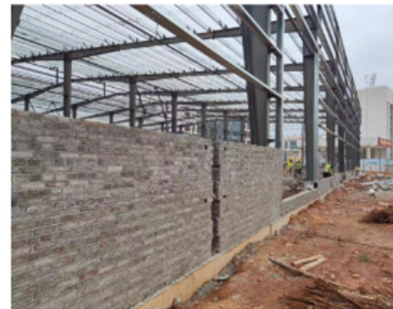
brick work at raw material workshop
