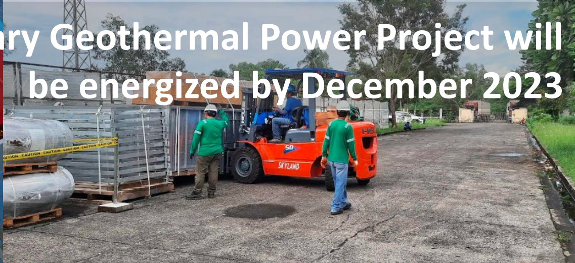
AIR COOLED CONDENSER COMPONENTS DELIVERY
