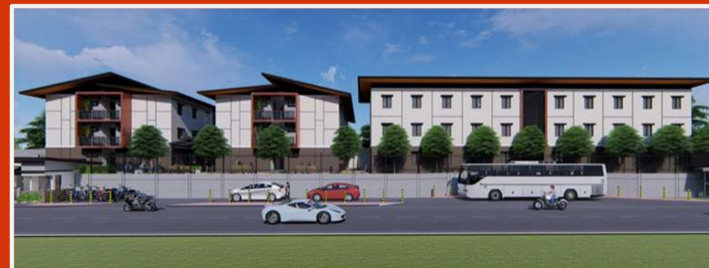
'The Pods' - LIMA's Dormitory Facility
