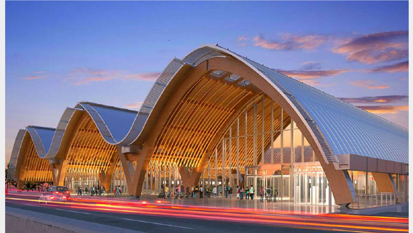
Mactan Cebu International Airport Terminal 2
