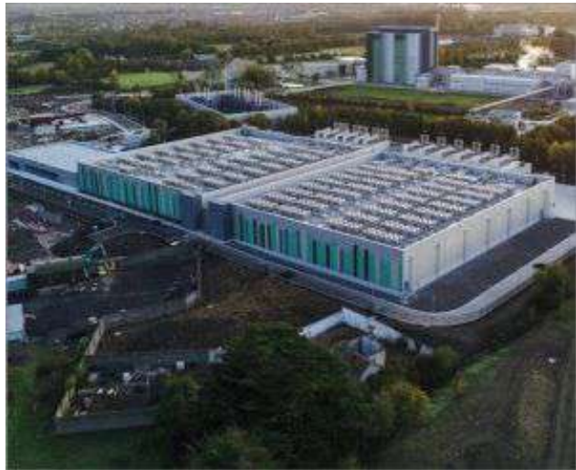
ECX Dublin Data Center
