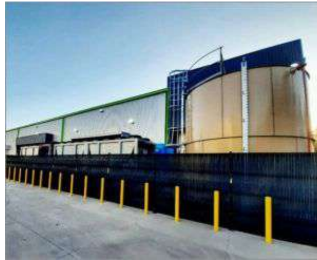
ECX Santiago Data Center
