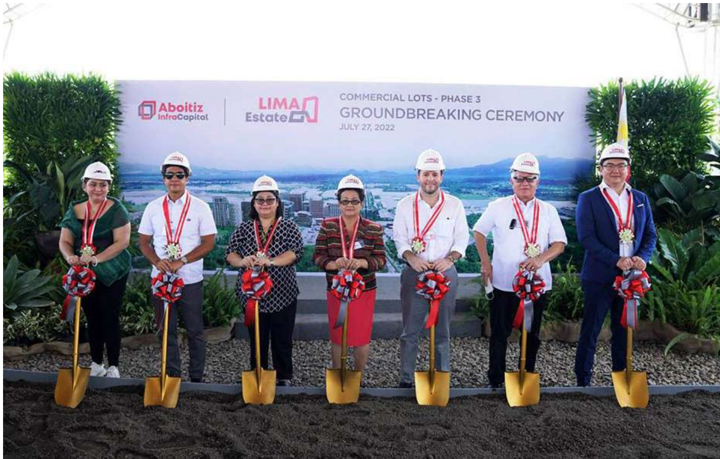
Groundbreaking for the third phase of commercial lots within LIMA Central Business District (CBD), the first master planned CBD in the province of Batangas
