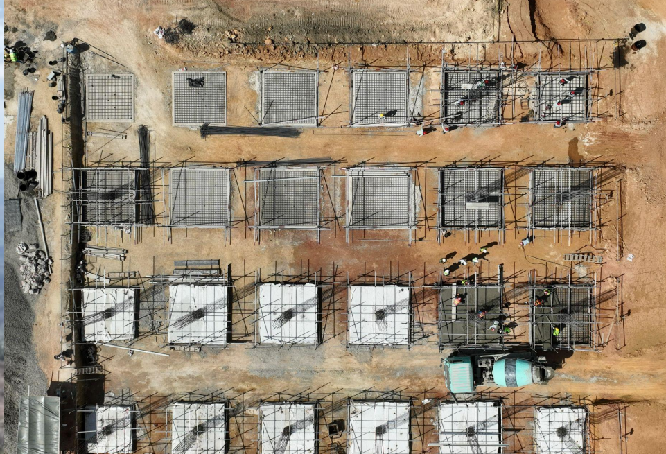
Rebar Installation and Footing Concrete Pouring Works for Powerhouse Foundation
