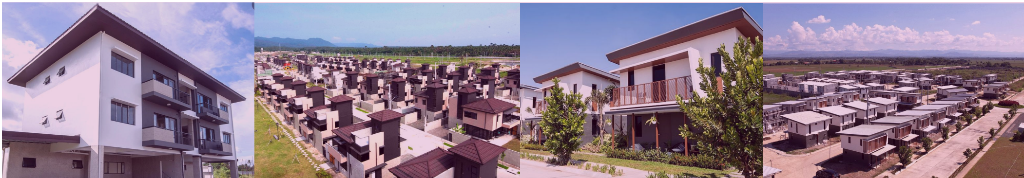
Construction showing significant improvement year on year
