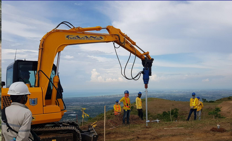
Screw Piling Works at PV Area
