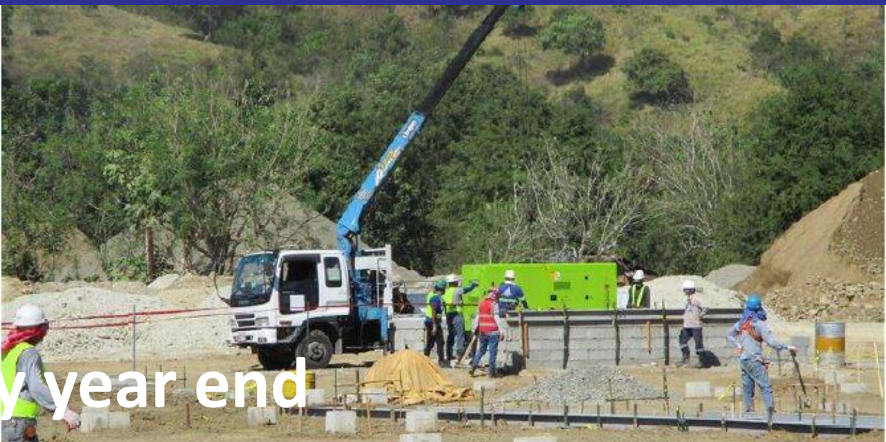
Temporary office pedestal installation
