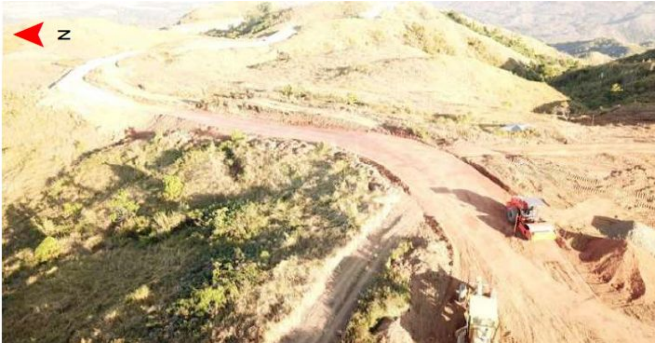
Road grading at PV plant site
