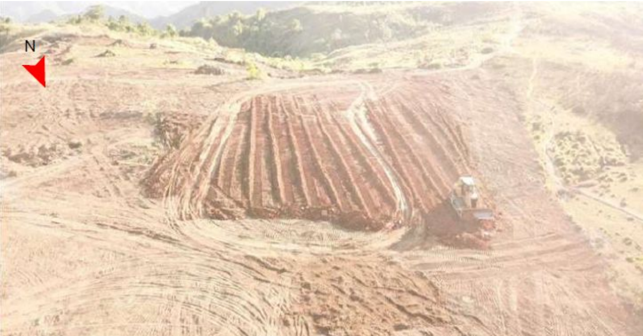
Grading works at the substation area
