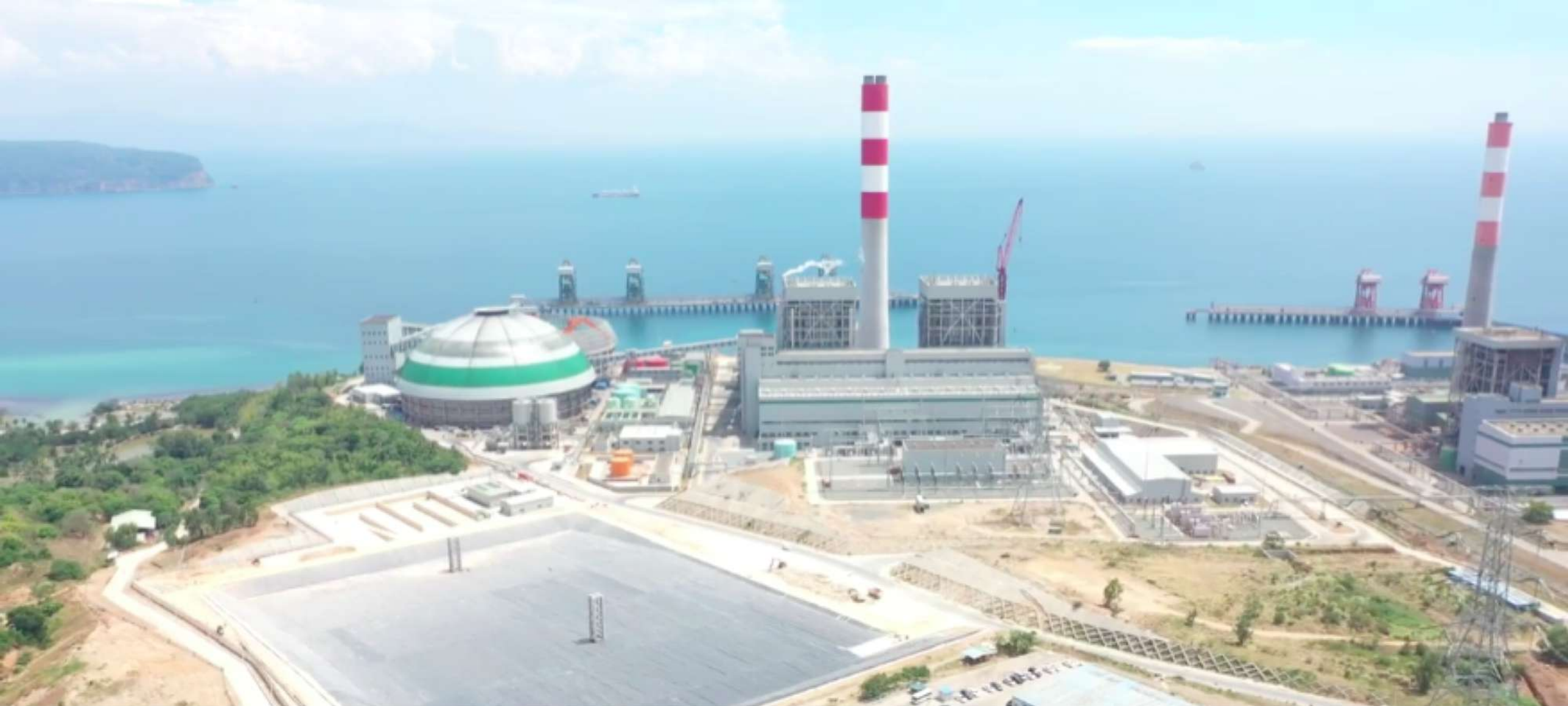
GNPower Dinginin 2 x 668 MW of Coal Power
