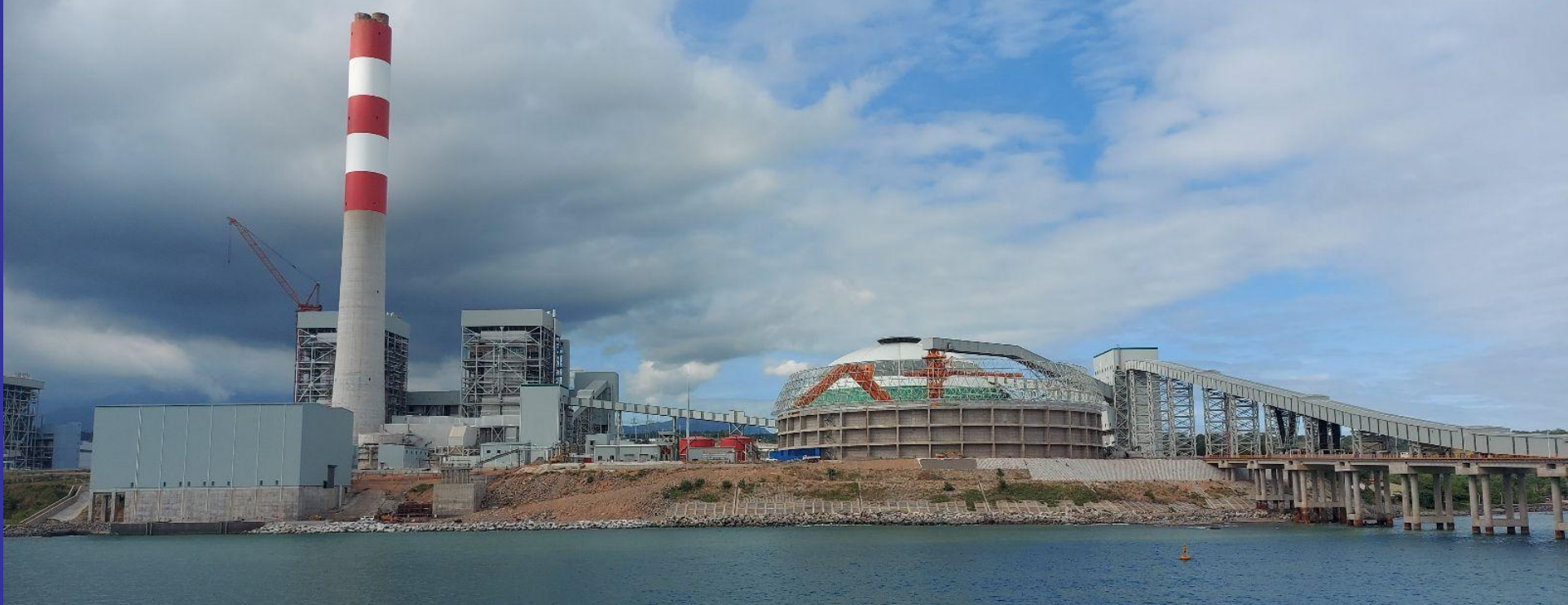
Plant View From Jetty
