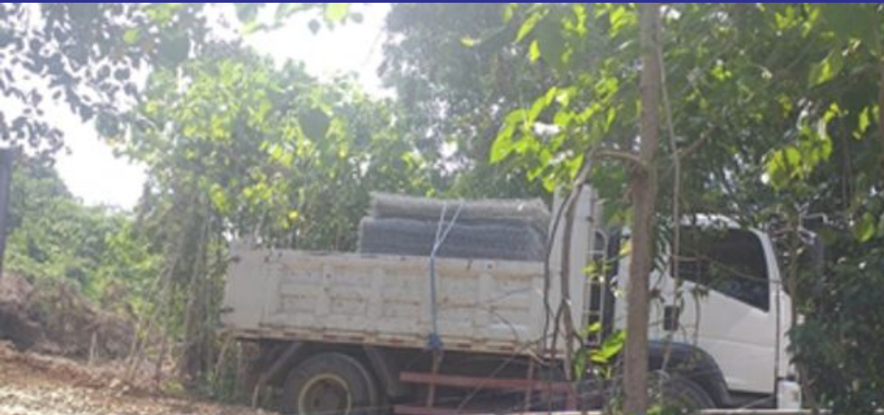
Delivery of slope protection materials
