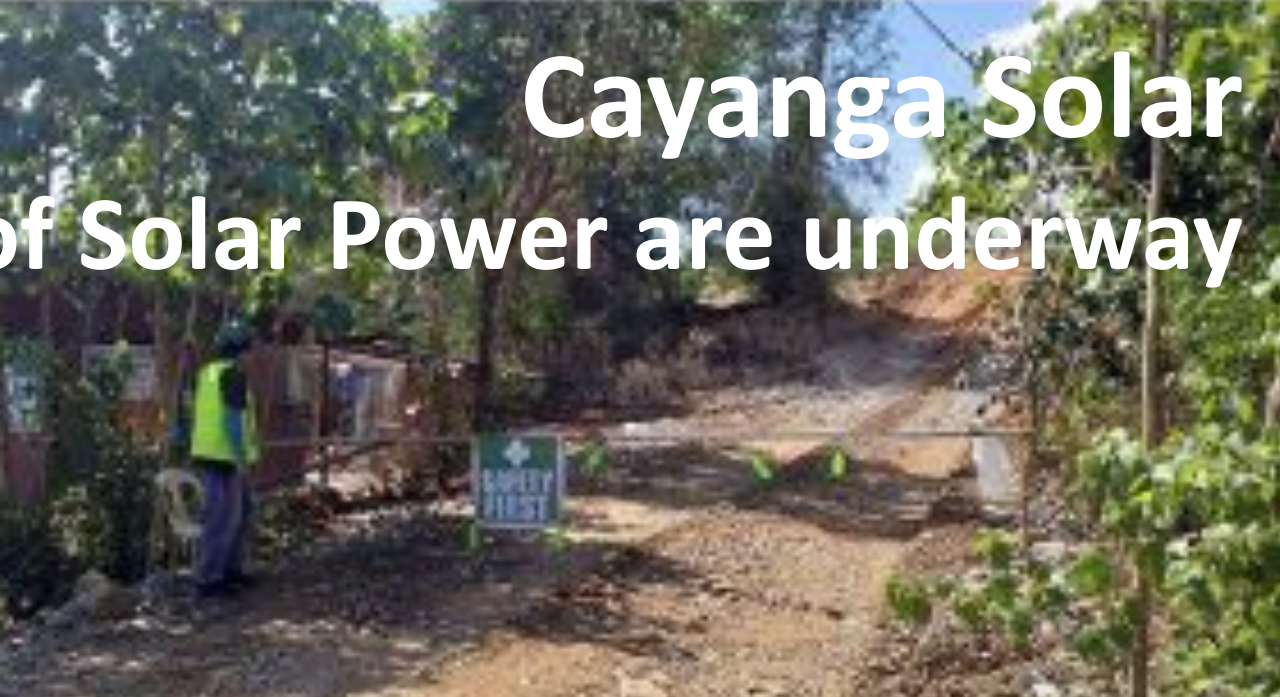
Establishment of temporary facility and guard post at site
