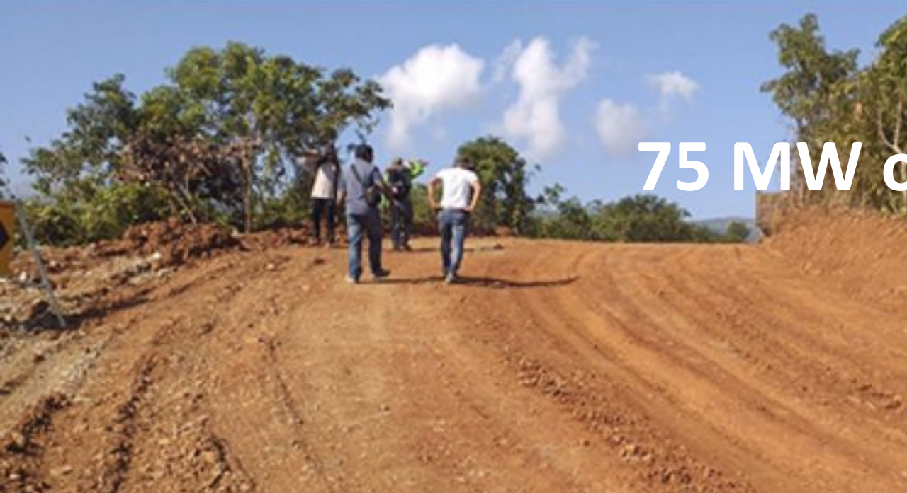
Joint inspection of excavation limits
