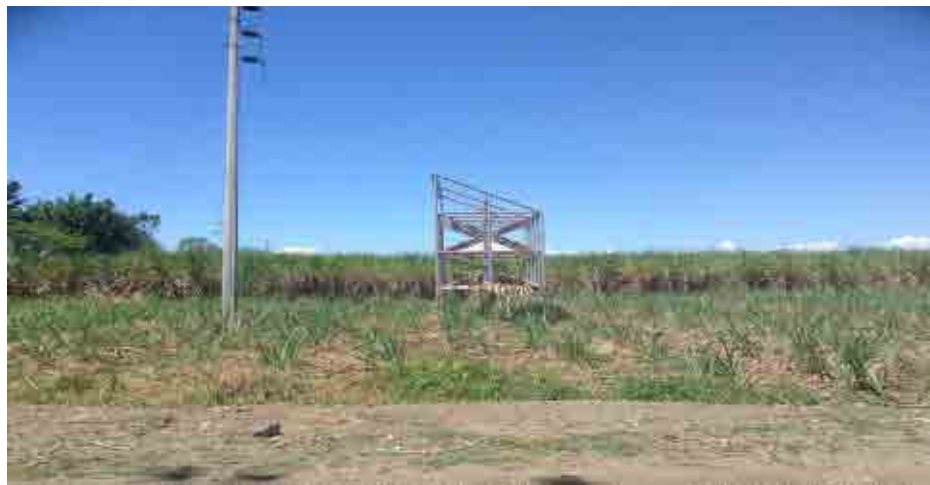
Image 6: South Side Near the Highway Facing North
