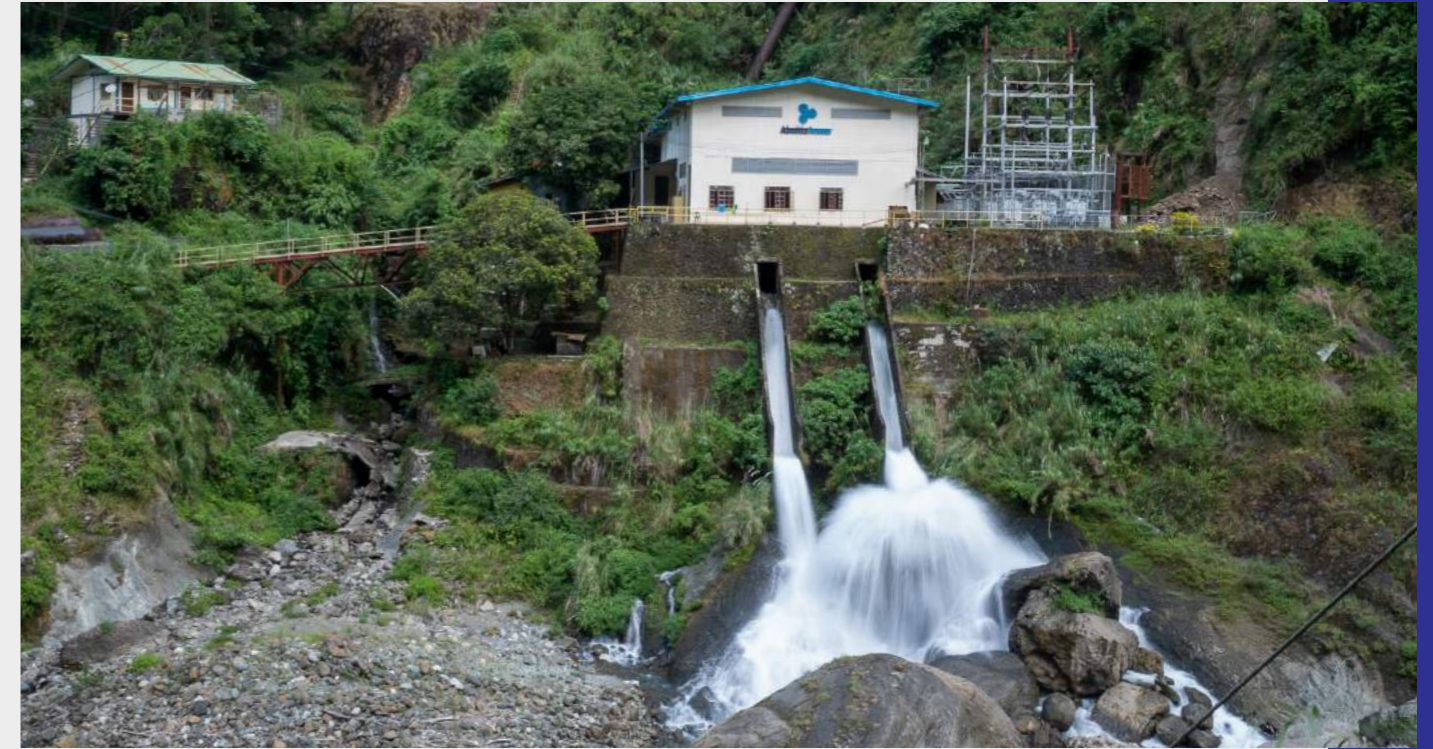
Hedcor's FLS Hydro (6.4 MW, gross capacity) located in Bakun, Benguet
